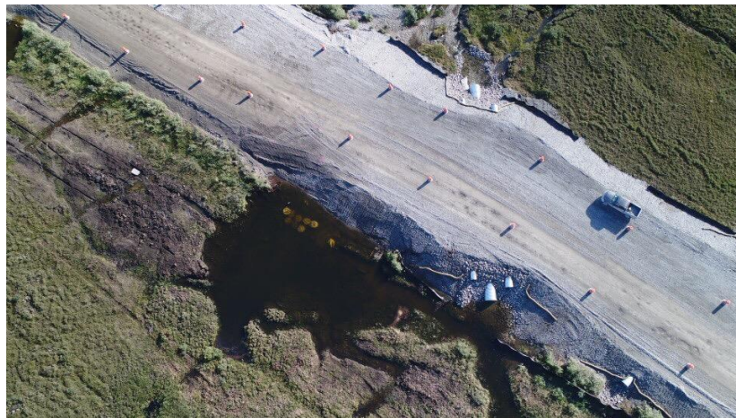
Impacts of impounded water along the Dalton Highway
