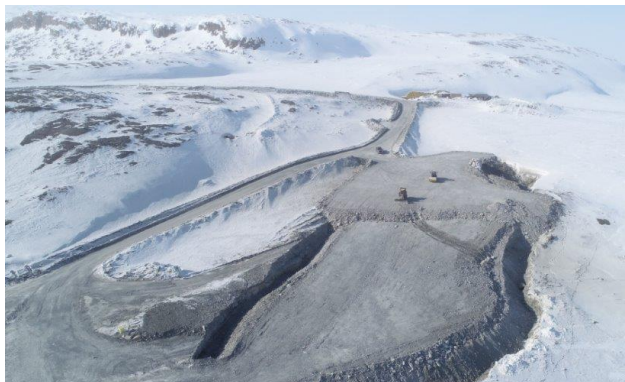
Run-of-mine backfill forming frozen cap over crown pillar in Nunavut
